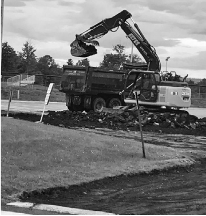
(Whitcomb's milling the old BTMES parking lot before putting down new pavement.)
